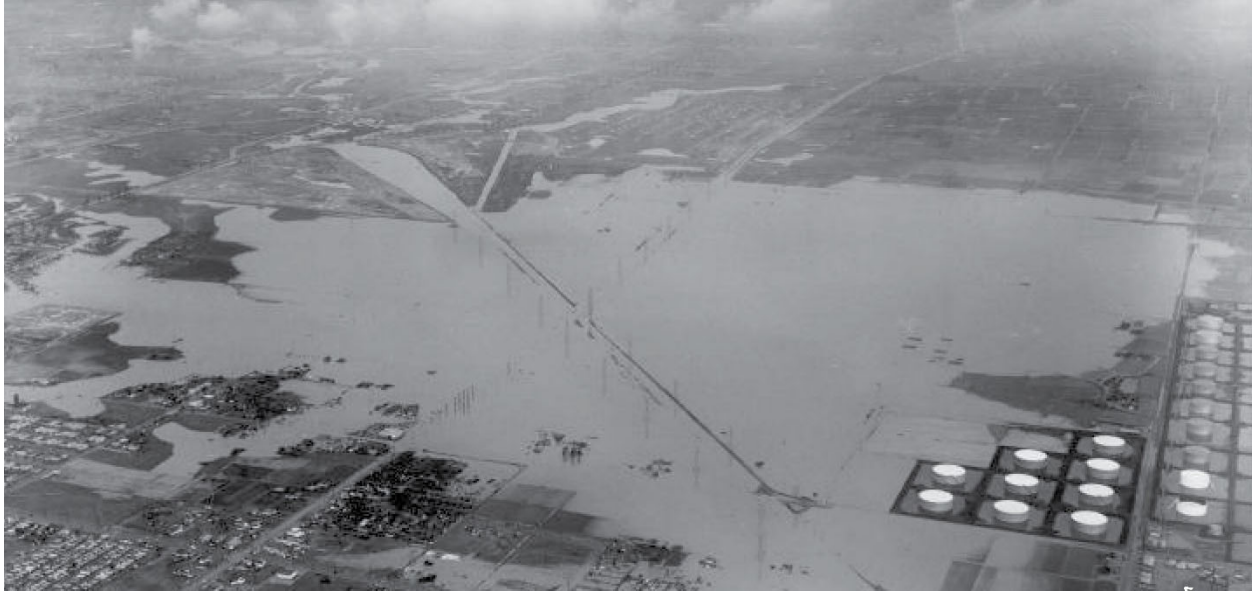
Source: Cal State Dominguez Hills, Aerial of Dominguez Channel Flooding at Present Day Victoria Golf Course, 1937.
