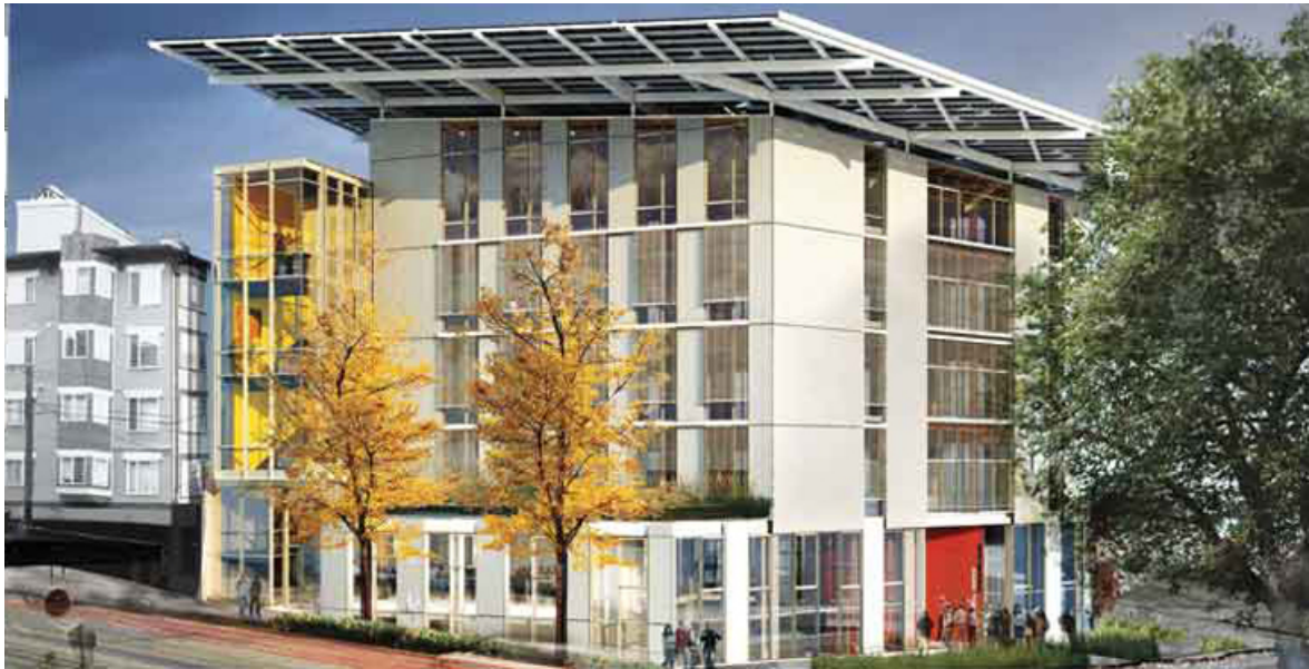
Figure 1- Bullitt Center, Miller Hull, Zero Net Energy (ZNE) building, Living Challenge building.
