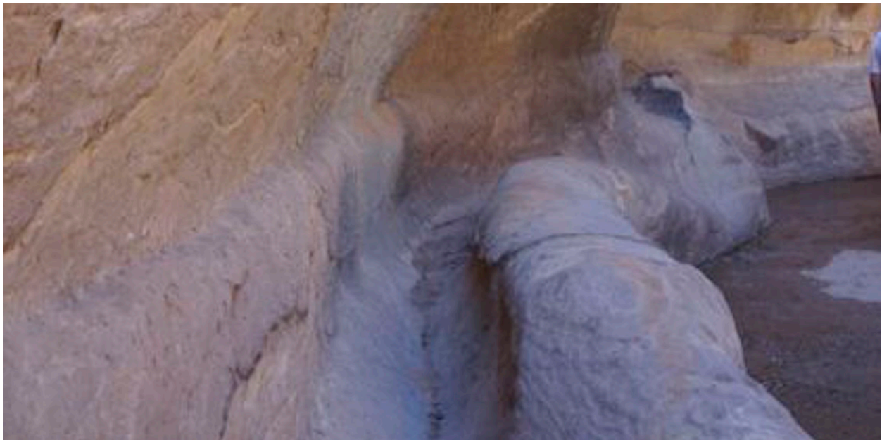
Nabatean sluice. Petra, Jordan. Photo by Hadley Arnold, 2015.
